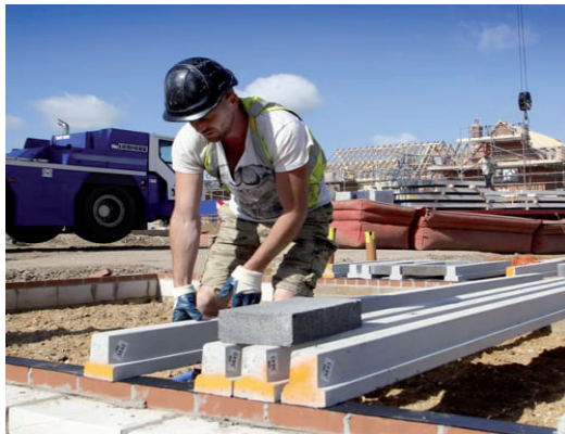
Poundfield Products manufacture high-quality precast concrete beam & block floors finished to a very high smooth standard
